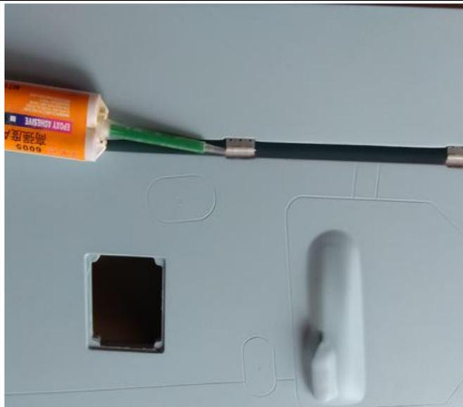
2. Epoxy the flap to the wing, Keep some space between the trailing edge and the flap to make sure it can rotate smoothly.
